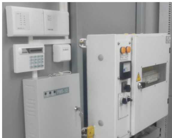
Fire alarm system
