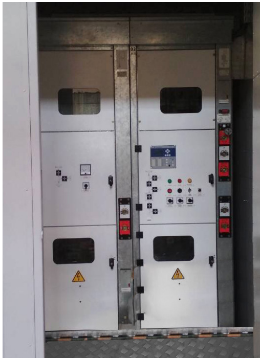
KSO-METZ-210 with vacuum interrupter
